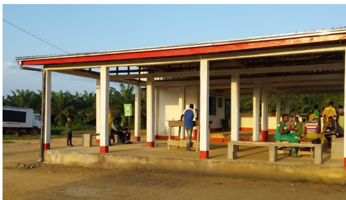
△ Hangar Commerces V3 Bis, Edéa, Socapalm
